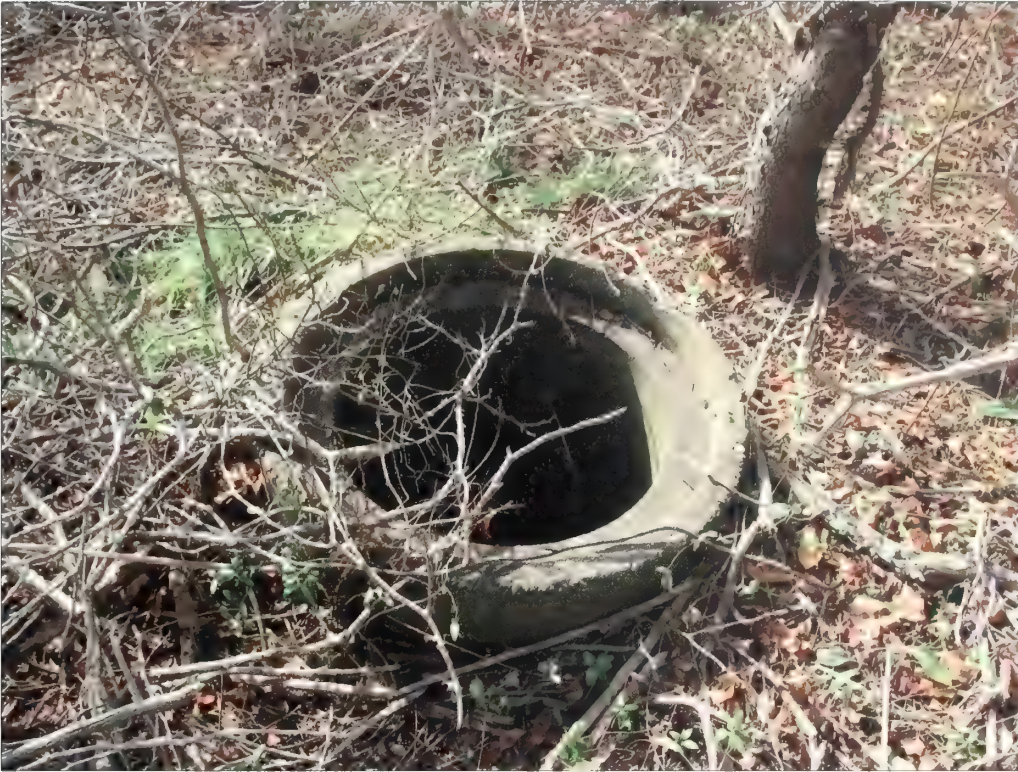
Figure 3.53. Concrete pipe, Battery Mills. Southwest of emplacement #1, a concrete pipe emerges from the engineered earthwork (Olmsted Center, January 2009).
